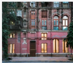
Gallery facade (night)
